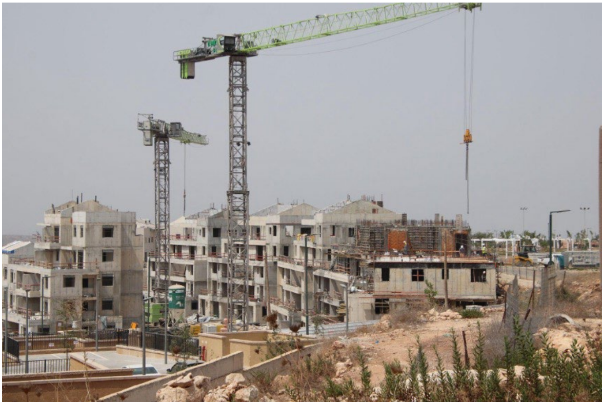
Construction site in Ofarim settlement.
