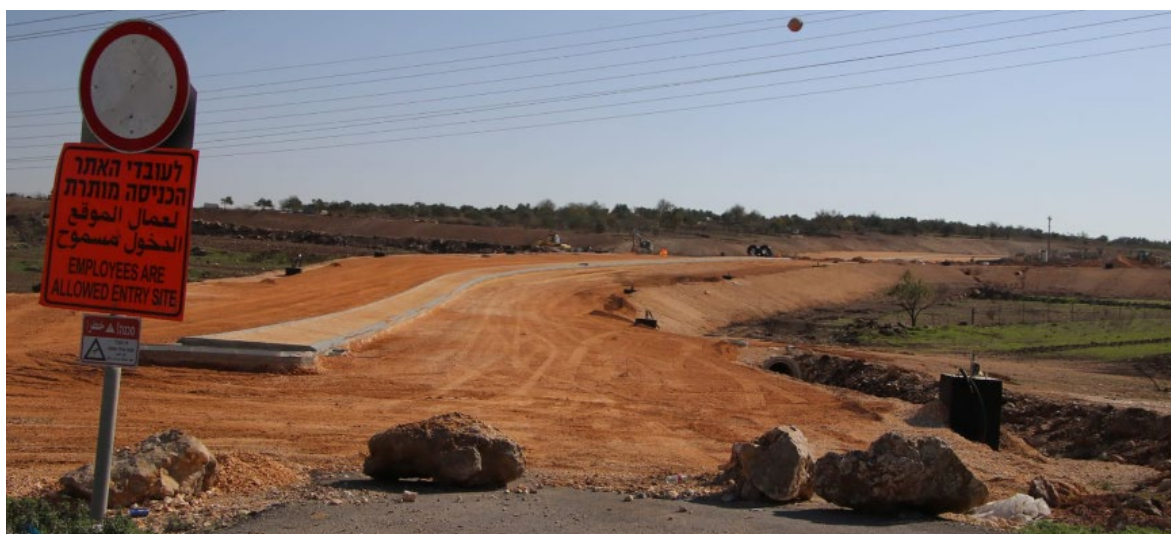
Construction work on the al-Funduq bypass road.
